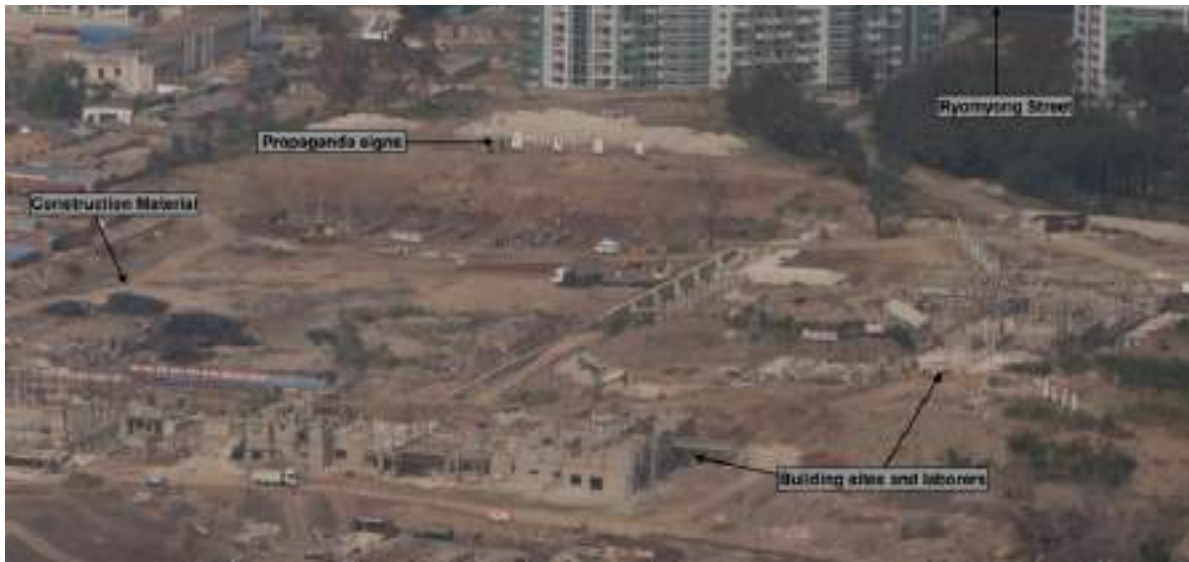
Figure 8. Close-up of Construction Site [Source: NK News]
